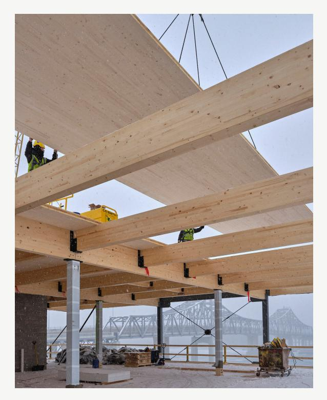
Mercer Mass Timber Building Solutions CLT/Light Frame
